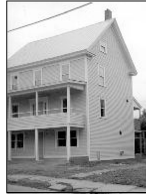
Figure 7. A six-bedroom rehabilitation in Gilman, Vt.
